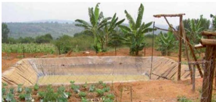
**Figure 1.** Rainwater harvesting pond.
